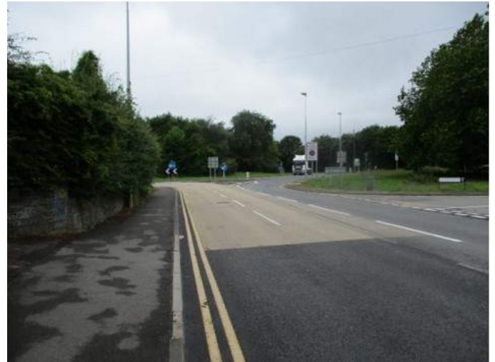
Highbeech roundabout westwards A48 access with new dual white line lane road markings
