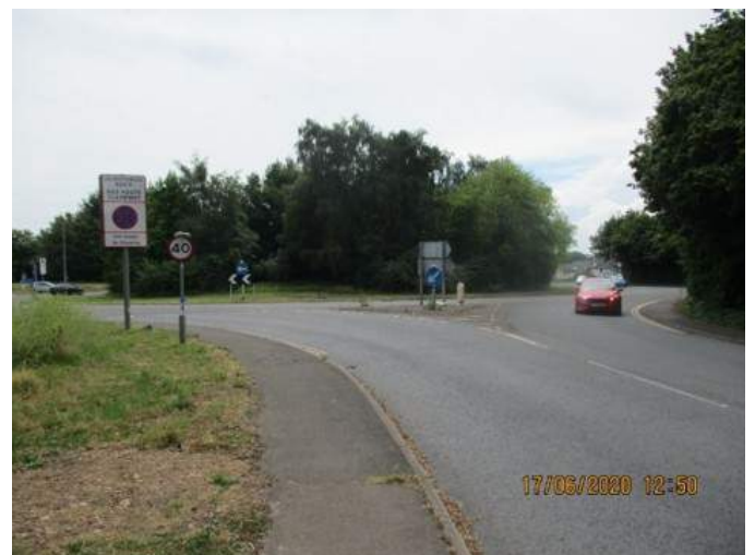
Highbeech roundabout southwards A466 access with NO dual white line lane road markings
